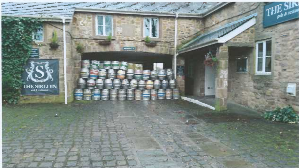
Entrance to car park blocked barrels, not a safe structure.
